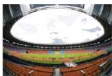
Main Stadium Gelora Bung Karno
